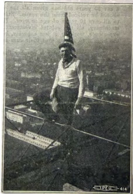
Washington, D.C., Local 26 wrote an article, attributed only to "The Crew," in the November 1934 Electrical Worker chronicling its members' work on the Washington Monument project. Above is Local 26 member E.A. Fritz at work on the project. This photo, along with the other photos accompanying this Grounded in History article, were printed in the November 1934 Electrical Worker.
