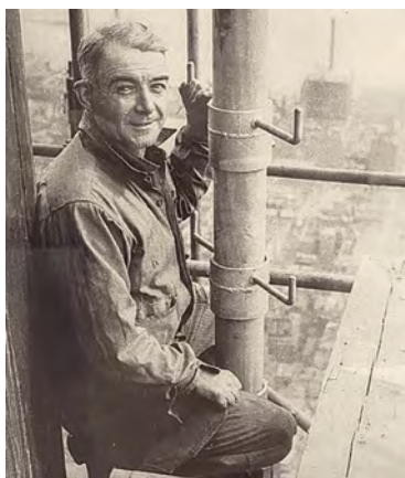
William Holmes, the grandfather of the letter writer, working on the Empire State Building. He was an IBEW member for nearly 50 years.
