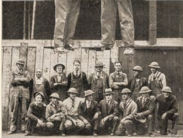
Falling debris at a jobsite in Boston in 1931 spurred the IBEW innovation of using military helmets as head protection
