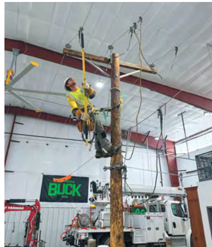
Apprentice Gunter Gosha of Local 702 training on EPZ grounding.
