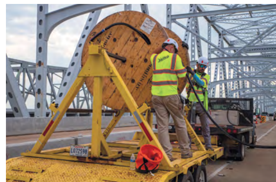
Field foreman John Bilich, left, and Local 130 apprentice Juan Gomez pull the primary feeders and feed the tray cable from the roadway to the catwalk below the bridge.
