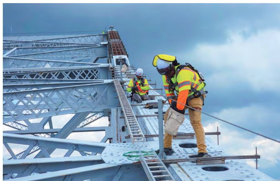
New Orleans Local 130 apprentice Shaun Rice, front, and journeyman wireman and field foreman Jaff Faulstich install cable trays on the support brackets to prepare for the installation of the necklace lighting wiring.
