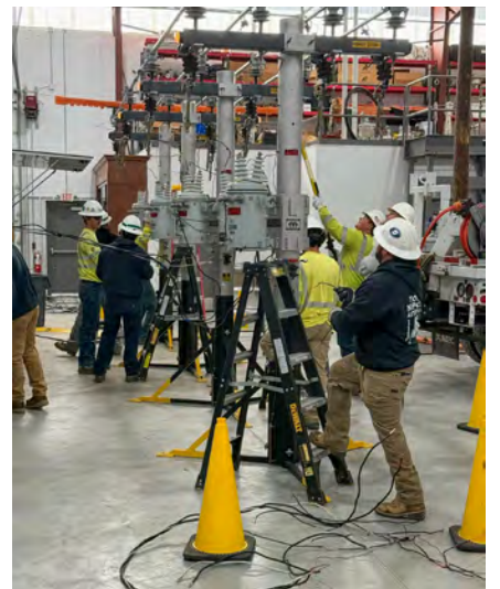
Local 702's transformer class gives apprentices practical experience in the assembly, maintenance and troubleshooting of transformers.
