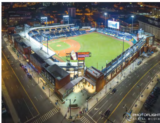
Local 35 helped build the Yard Goats' baseball stadium in Hartford, Conn.
