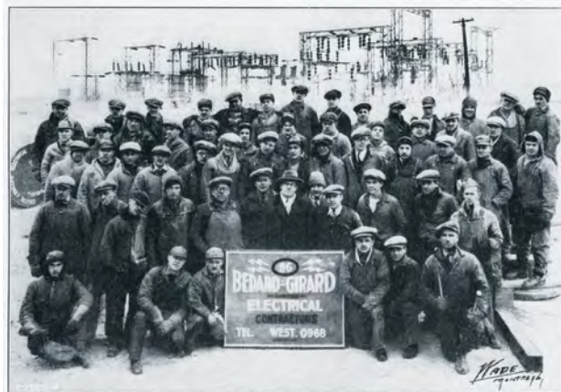
MONTREAL LIGHT, HEAT AND POWER CONSOLIDATED SUB-STATION AT MONTREAL, EAST. 100 PER CENT UNION JOB BY MEMBERS OF L. U. NO. 568, I. B. E. W.
