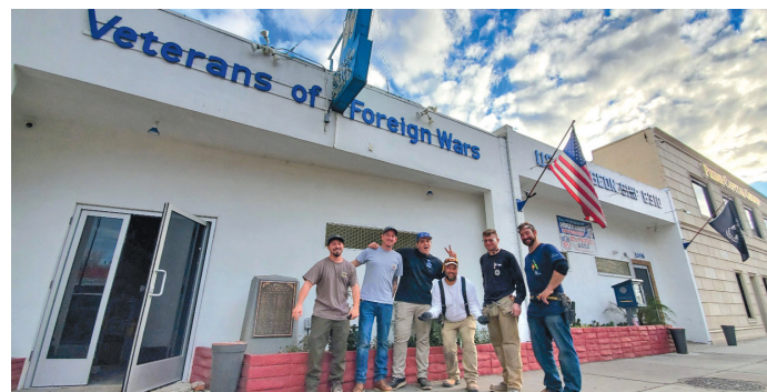
Local 40 RENEW Committee members helped with a complete rewiring and new light install at the Veterans of Foreign Wars in Burbank, CA.
