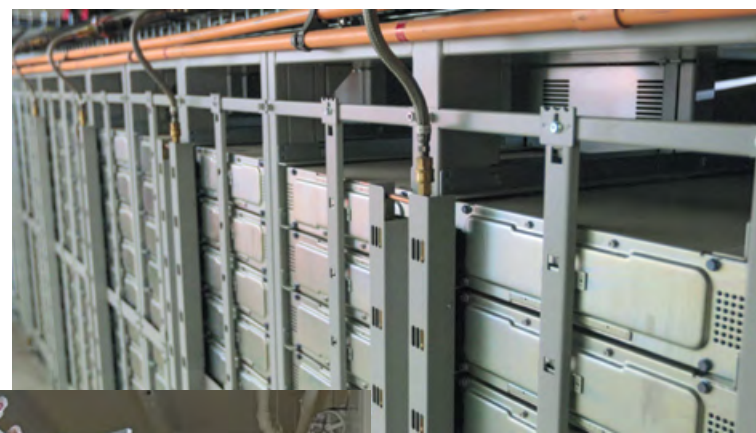
Local 234 members installed nearly 100,000 batteries, 22 in each rack, weighing nearly 12,000 tons in total.
