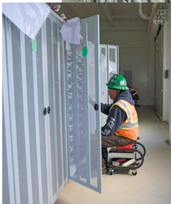
Local 234 members installed nearly 100,000 batteries, 22 in each rack, weighing nearly 12,000 tons in total.
