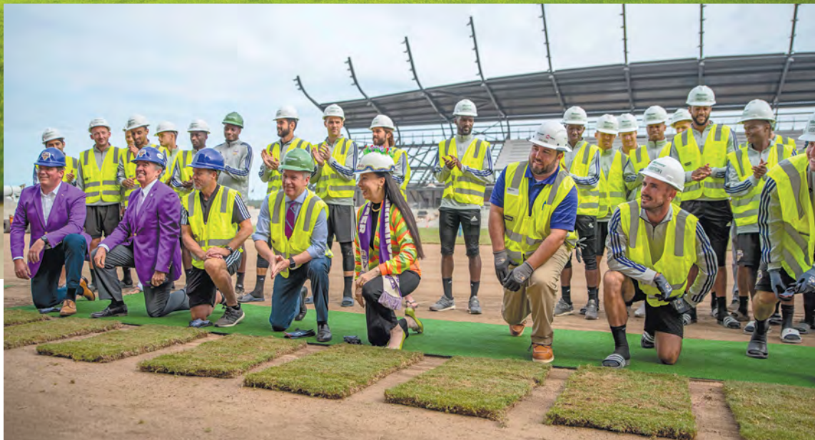
More than 60 Louisville, Ky., Local 369 electrical workers installed everything from wiring to signs at the city's new soccer-only Lynn Family Stadium, where Louisville City F.C. officials and players joined construction officials last summer to present samples of natural grass turf to be used there.
