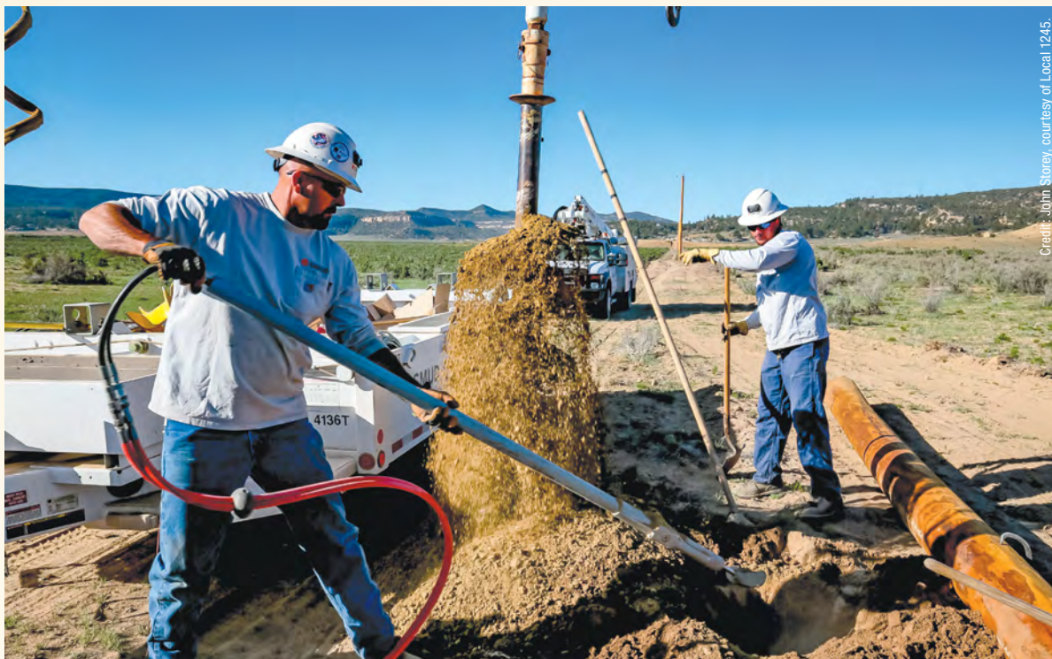
Above: Kevin Cranford, left, and James Cotton, dig a hole for a new pole. The Vacaville, Calif., Local 1245 members were part of a five-member IBEW crew from the Sacramento Municipal Utility District who spent two weeks in the Navajo Nation in April and May 2019. Right: Their Local 1245 brother Corey Smith in a SMUD line truck.
