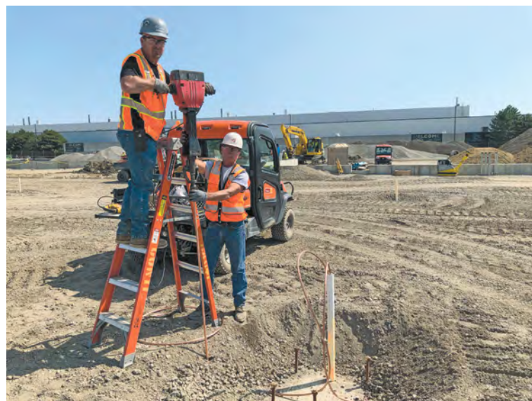
Top: The cleared site of Fiat Chrysler's Mack Avenue Assembly Complex as construction began and a rendering of the finished complex. Above: Detroit Local 58 members Scot Bishop and Bill Volkman installing substation ground on the site of the first new auto plant in the city for nearly 30 years.
