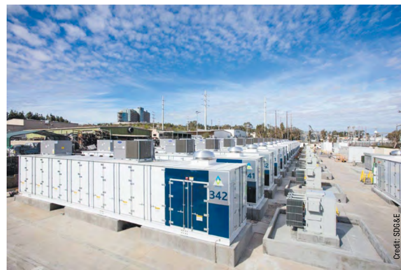
The 30 MW Escondido (Calif.) Storage facility, built by members of San Diego Local 569, is part of the more than 1 GW of grid storage needed to stop utility carbon emissions in the state by 2045.
