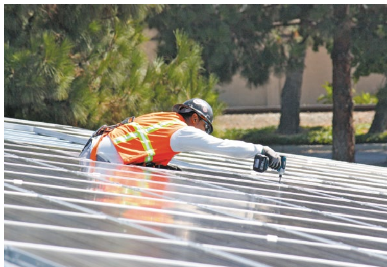
Together, these new organizing tools will redefine the way we bring new people into the IBEW, brightening the work picture for every member.
