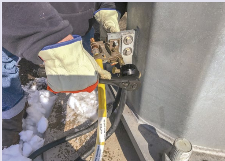
Ground clamp bolts come in all shapes and sizes; now one tool turns them all.
