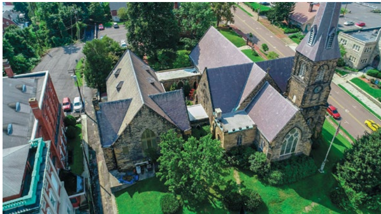
Wiring upgrades by Cumberland, Md., Local 307 members will help protect the historic Emmanuel Parish of the Episcopal Church, which once served as a stop on the Underground Railroad.
