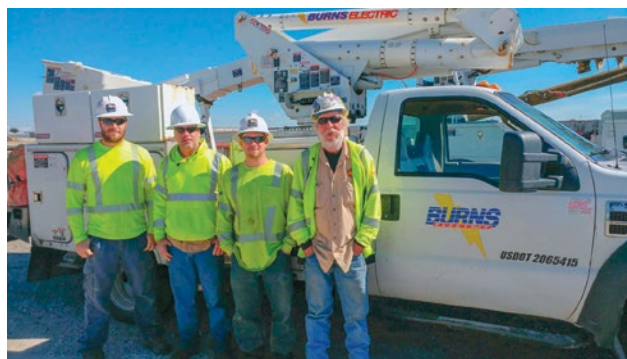
Local 55 crew working for Burns Electric on a cost-plus job for Story City Municipal Electric Utility. From left: Nick Dougherty, Chris Lichty, Andy Brodahl and foreman Brian Opstvedt.
