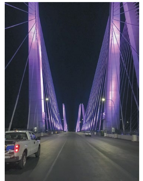
Local 363 extends new year’s greetings from the Rockland, NY, side of the new Gov. Mario Cuomo Bridge, which replaces the old Tappan Zee Bridge.
