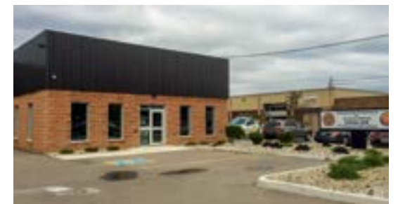
New IBEW Local 530 union hall opened on Oct. 23, 2018.
