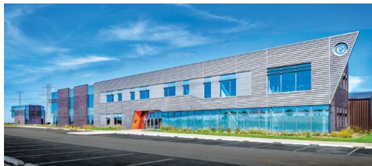
A decade in the making, Chicago Local 9's new University Park training campus was designed to be flexible enough to serve an evolving electrical industry.
