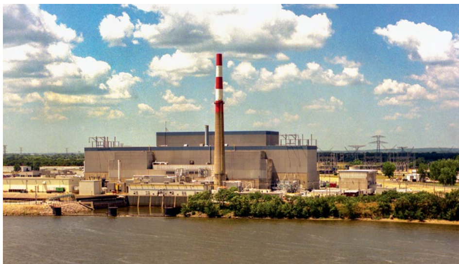
The Quad Cities nuclear plant was scheduled for closure until Illinois passed a support system for non-carbon emitting power generation.
