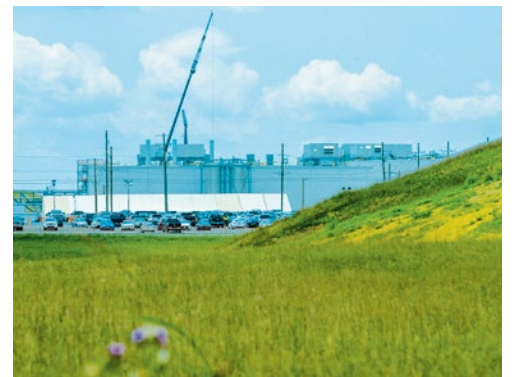
The $500 million Procter & Gamble plant in Inwood, W. Va., will create thousands of jobs both during and after construction.
