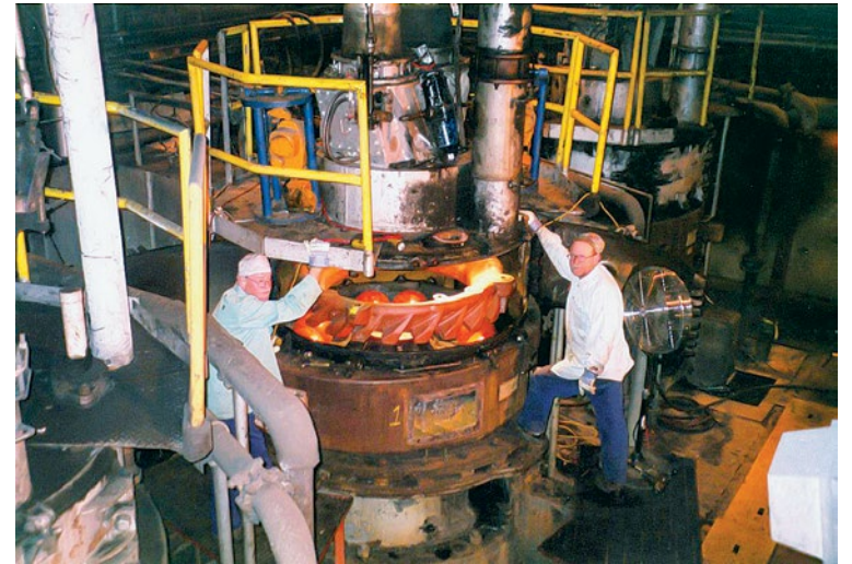
West Frankfort, Ill., Local 702 members working on one of the final overhauls before unit #1 shutdown at the Culley Generating Station in southern Indiana. Photo by Elizabeth Weyer
