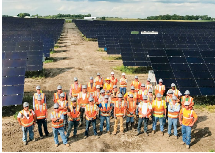
Local 292 members are busy with work on solar farm projects.
