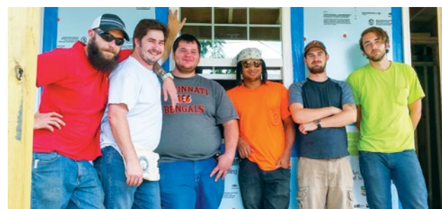
Local 212 RENEW volunteers wire Habitat for Humanity houses. From left: Michael Sansone, Richard Heimbrock, Joseph Knapp, Andrew Daniel, Kaleb Burkhardt and Ernest Spencer.
