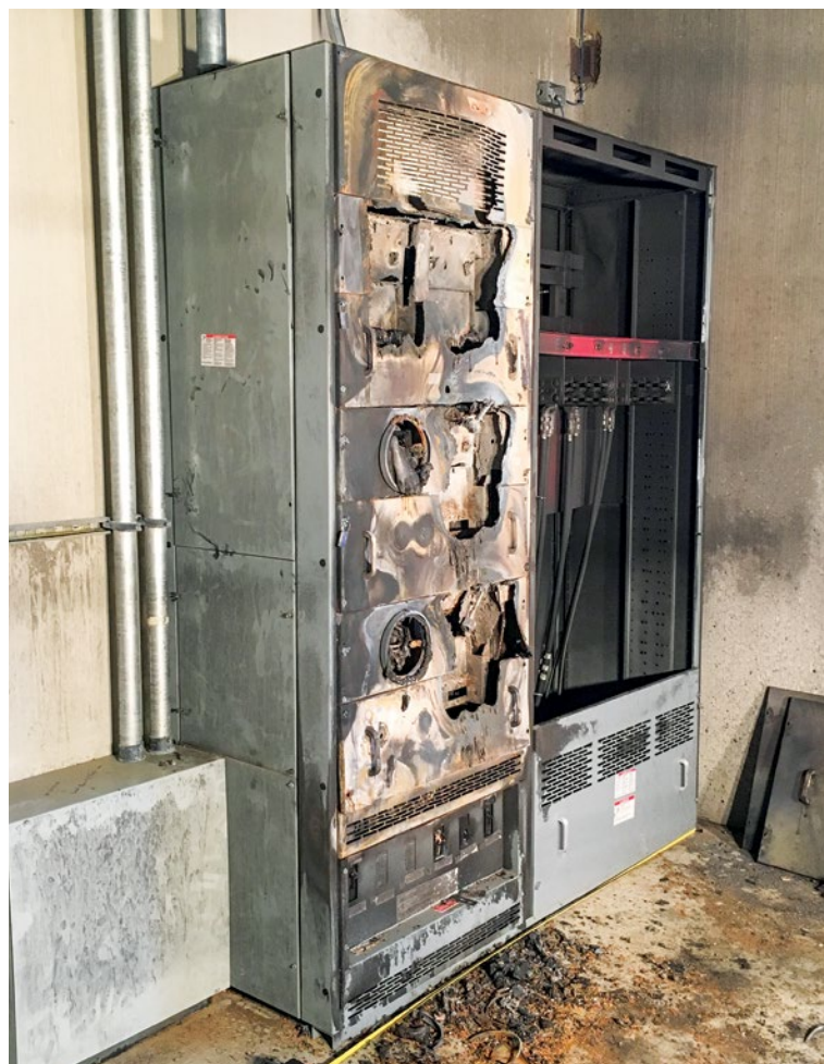
Portland, Ore., Local 48 journeyman wireman Jeremy Sells was kneeling in front of this panel when it arced, repeatedly, melting the front of the switchgear and spraying him and his tool cart with molten metal shrapnel, shown at top.
