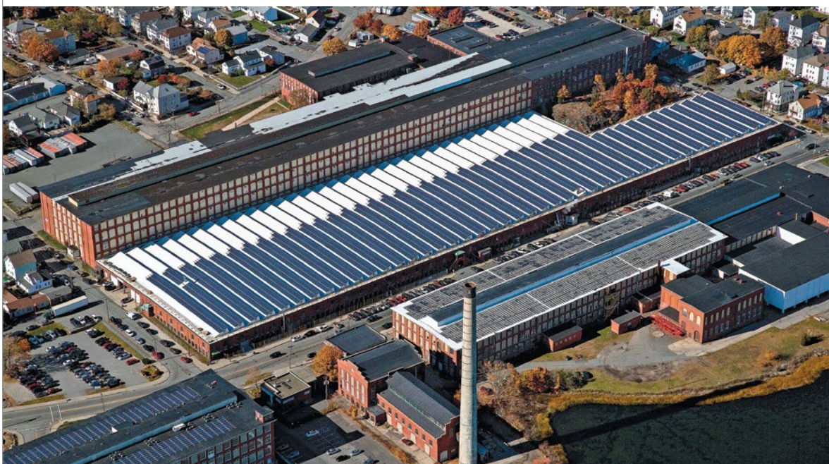
IBEW members working for Beaumont Solar built the 1.3 megawatt rooftop solar system on the union Joseph Abboud suit factory in New Bedford, Mass.
