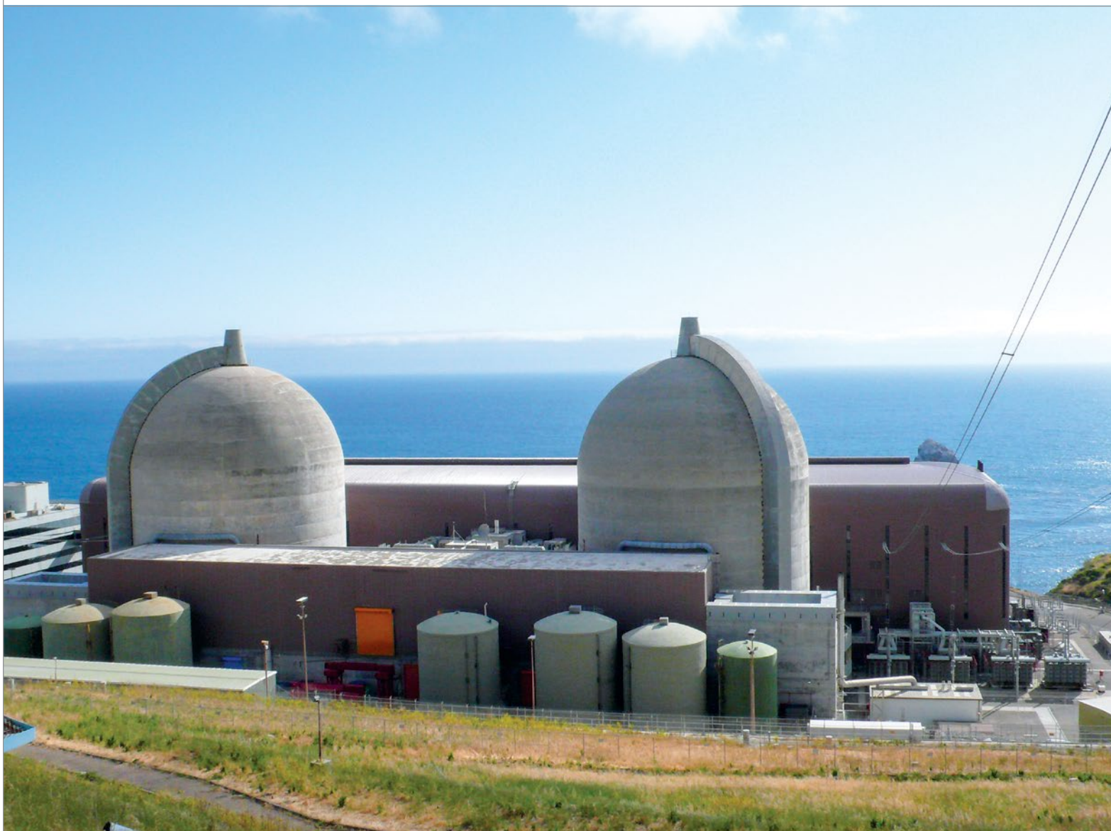
The Diablo Canyon nuclear plant sits on a cliff overlooking the Pacific Ocean. In 2025, it is slated to close, leaving the state without nuclear power for the first time since 1957. Photo used under a Creative Commons license from Flickr user bikracer.
