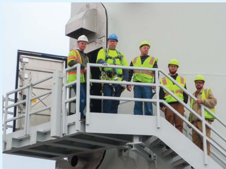
Local 99 members Chris Seiber, Chris Wilson, Jonathan McKeen, Jon MacDonald and Matt Lattinville assemble before they enter a wind turbine tower to perform insulation work.
