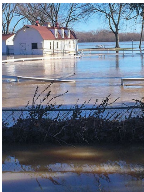
View of December 2015 flood damage at Ride On St. Louis site in Kimmswick, MO. (Photo courtesy IBEW Local 1 and Ride On St. Louis.)
