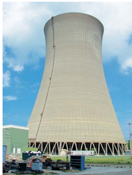
Unit One cooling tower at the Perry Nuclear Power Plant in Ohio.
