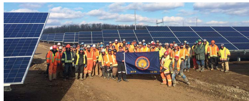
Hamilton, Ontario, Local 105 members on the Grand Renewable Solar Project in Cayuga.
