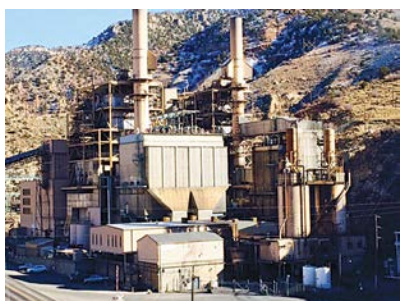
The coal fired steam generating plant that employs Local 57 members will soon undergo a decommissioning process.
