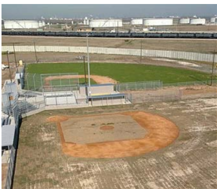
Beaumont, Texas, Local 479 apprentices volunteered their time to build a new Little League field.
