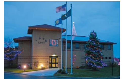
IBEW Local 99 holiday lighting display installed at union hall.
