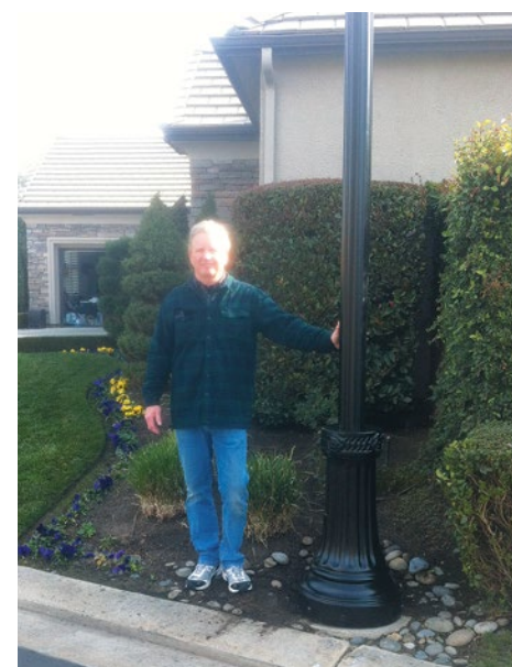
Local 100 retired Bro. Brad Ballenger stands beside a new light pole at his house, installed by Electric Motor Shop.
