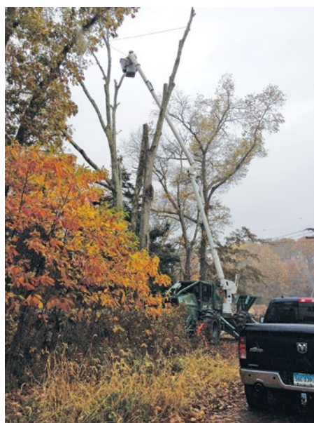
Local 42 "BA" members perform tree clearing along distribution rights-of-way.
