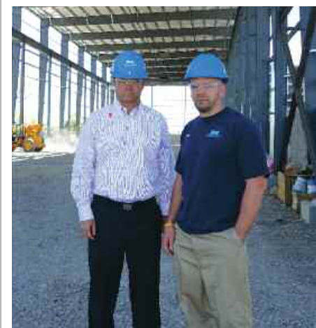
Owner John Darby (left) and Local 41 Steward Ron Bailey stand in front of Niagara Transformer's building expansion.
