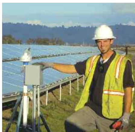
Daniel Gilbertson, Local 234 fifth-year apprentice, checks the weather station at the 222.5 KW solar array at Watsonville Water Resources Center.
