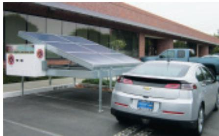
IBEW Local 332 solar-powered charging station for electric vehicle.
