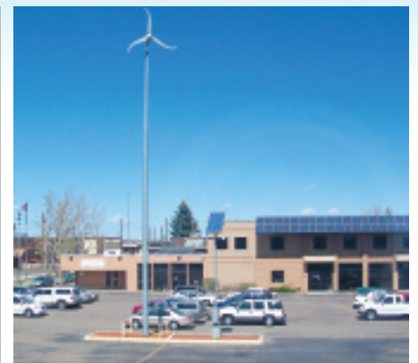
Wind turbine and solar panels at Denver Local 68 union hall.
