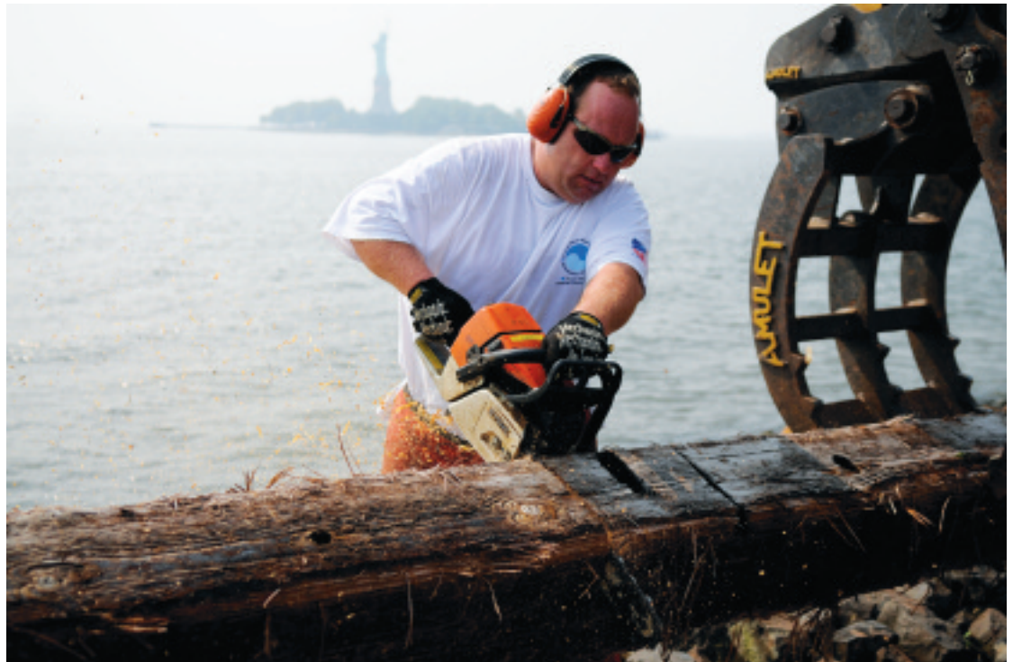
Members of Newark, N.J., Local 1158 supported the establishment of a Code of Excellence to showcase their skills at the Passaic Valley Sewerage Commission's facility, one of the nation's oldest and largest sewage treatment plants.
