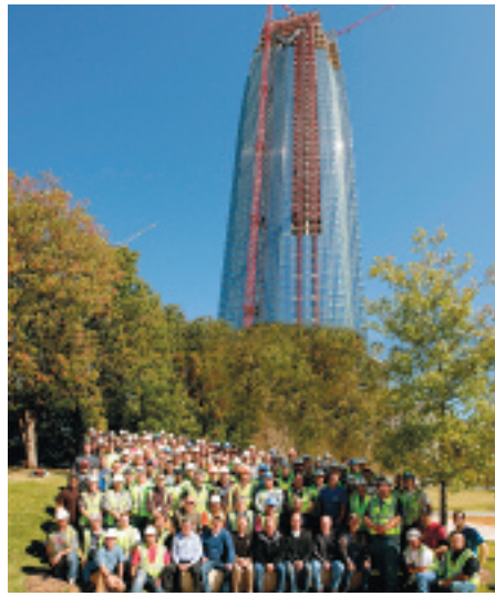
Nearly 200 members of Oklahoma City Local 1141 are building the new Devon Energy world headquarters—the tallest skyscraper in the Sooner State.
