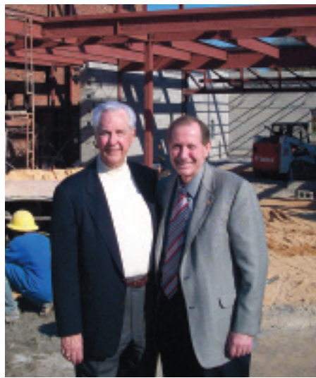
Bus. Mgr. Ken Ward (right) and Int. Pres. Edwin D. Hill visit the IBEW Local 1579 Training Facility construction site.
