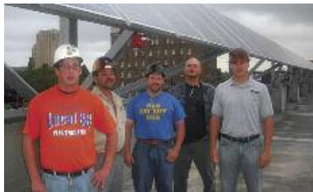
Local 38 members installed a new Cleveland State University solar array system. From left are: Mike Juliani, Craig Hurley, Jeff Rudy, Jarrod Amberik and Tom Grabowski working for Ullman Electric. Shown in the background is the new $40 million CSU student center being wired by IBEW members with Lake Erie Electric.
