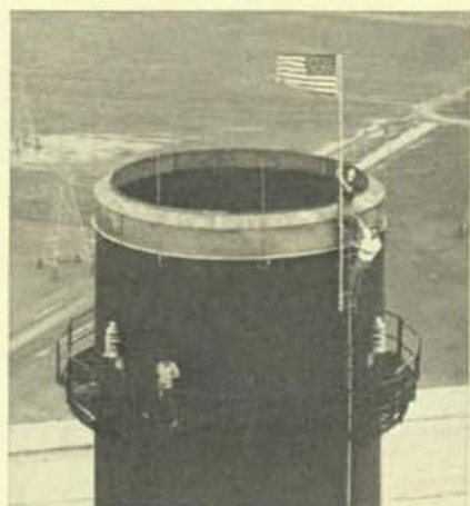
On Memorial Day, members of Local 1, St. Louis, climbed the 700-foot smokestack of Union Electric's new generating facility at Labadie, and affixed the American flag to the top. Shown here are Brothers Bob Taylor (at top of stack), Ed Garcia (on ladder), and Jim McNulley, who is loading his camera to take pictures.
