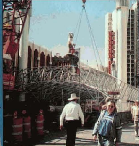
Crane begins to lift canopy skyward.
