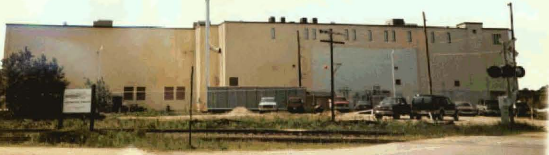
The 100-percent-union-built Virgin Pulp Substitute Facility in Auburn, Maine.
