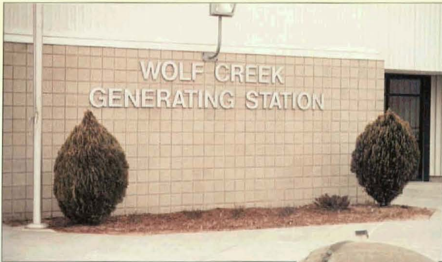
Front and rear view of the massive Wolf Creek Nuclear Plant.
