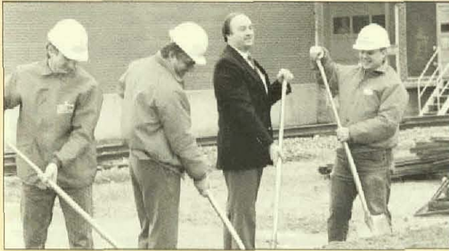
James Peplinski (far right), Local 1147, Wisconsin Rapids, Wis., steward, takes part in groundbreaking for the Consolidated expansion.
