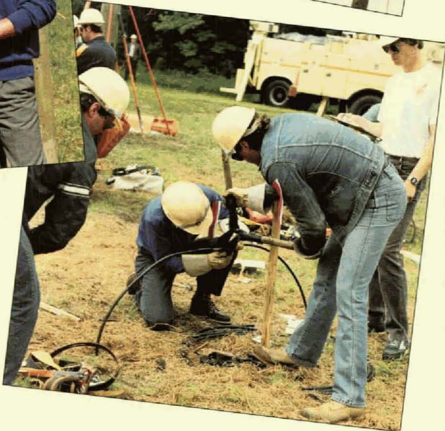
A team performing secondary splicing.
