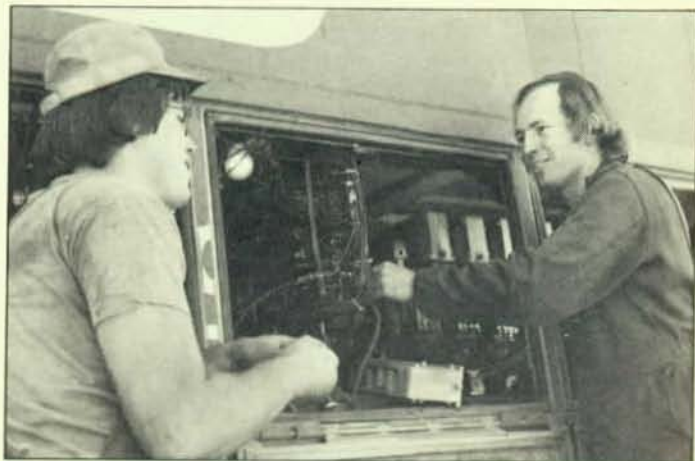
Apprentice S. W. Liggett (left) and electrician L. F. Fry check out diesel electrical cabinet at Burlington Northern's new multi-million dollar maintenance facility at Alliance, Nebraska.
