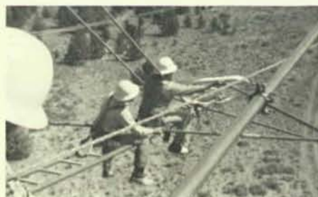
These photos show Portland General Electric crews learning to do 500-KV hot-stick work. Many of the employees had never done any hot-sticking on 500-KV. (Photos submitted by Local 125, Portland, Ore.)
