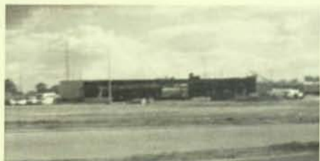
New HyVee grocery store under construction near the shopping center site.
