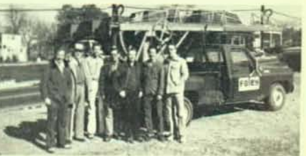
Local 26 electricians donate their time to install Christmas decorations for the city of Gaithersburg, Md.
