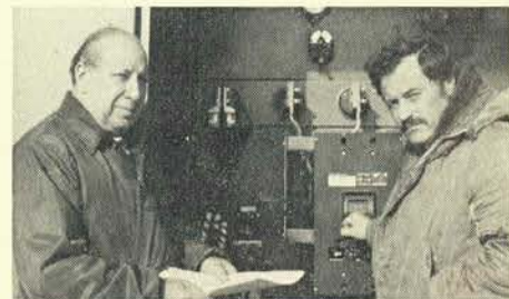
Contractor Harry Sassaman and general foreman Jack Connolly checking out equipment.
