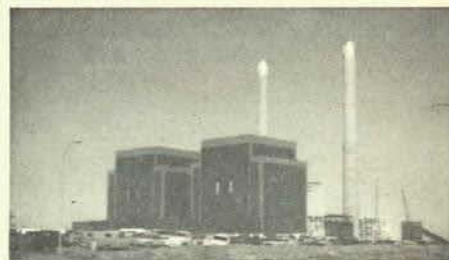
Unit I and II being built by the IBEW.
