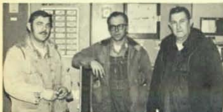
Shown in front of some switchgear at the plant are, left to right, Brothers Dick Bouma, Armand Sheffield, and Jess Ferguson.
