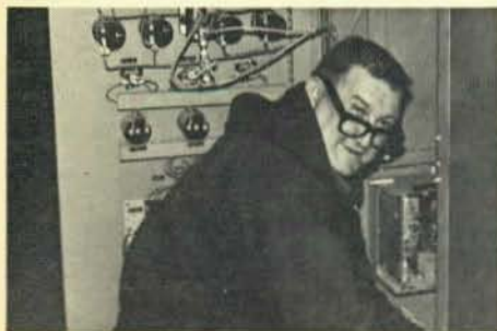
Brother Jess Ferguson making up switchgear at the sewage treatment plant.
