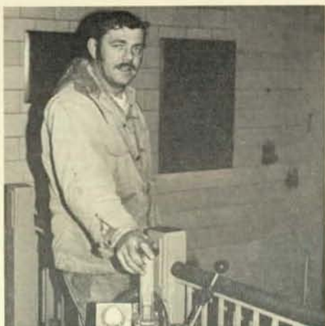
Brother Dick Bouma preparing to core-drill some holes.
