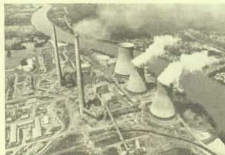
This picture of the John E. Amos power plant was taken while the No. 3 unit was under construction.
