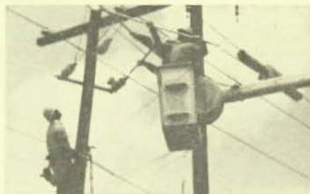
Local 398 linemen on the job.
