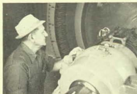
Brother Joe Tomasini, maintenance electrician, inspects brushes on the generators at Deerfield number four station.
