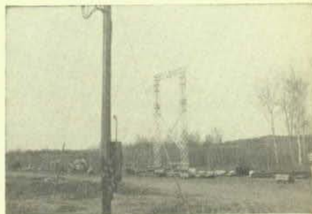
This is the aluminum structure for D.C. 500-KV line from Center, N.D., to Duluth, Minn.
