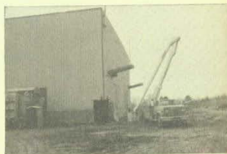
The outside of the D.C. converter building.
