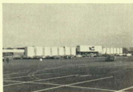
Part of new Chatham Place Mall.
