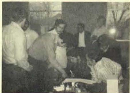
More Brothers work on 15-KV splice.
