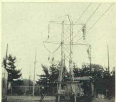
Training tower located in Hicksville Yard.
