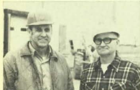
John Moreland and Hurschel Clements, both employed by Price-Fewell Electric Company, work on Speed Queen Washing Machine Manufacturing Company addition at Searcy, Ark.
