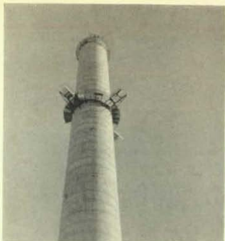
Local 231 members work at these sites. Shown here is 425-foot chimney at Port Neal Generating Station; photo is by Brothers Jim Cummings and Bob Lane, who installed lighting.
