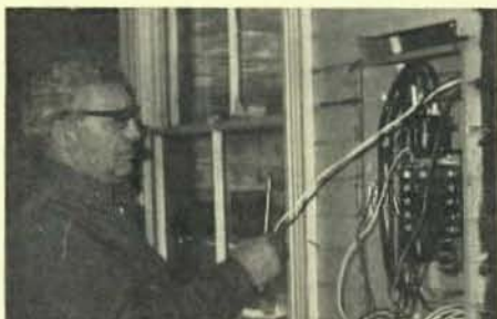
Local 806 President Sal Accardi cutting in panel at new local offices.
