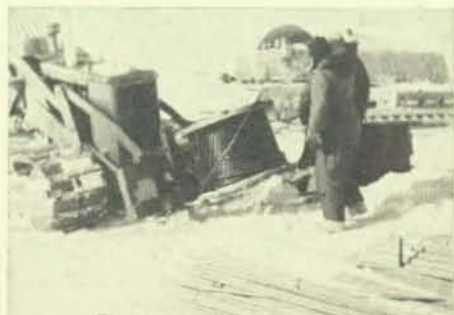
Brother Wolff, foreground, helping to load cable.
