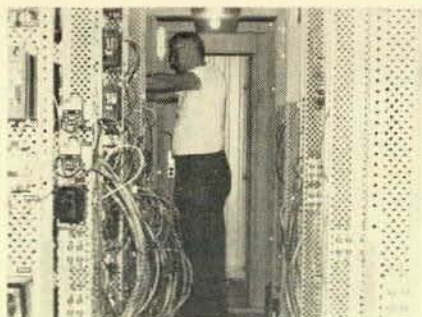
Brother Fred Wrezesien doing panel in tunnel substation.
