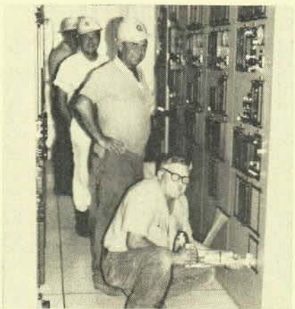
Brothers Brochu, Cone, and Nuhfer on the tunnel job for Carter Electric.
