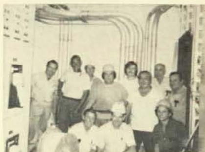
These members of Local 130, New Orleans, La., are building a new TV station for WVUE-TV. Kneeling, left to right, are steward J. Hennessey; Glen Hill of Local 1139, New Orleans, who coordinated the work for WVUE; and A. Zucconi. Standing, E. Montague, F. Schmitt, foreman E. Carver, Sr., E. Carver, Jr., J. Guidry, C. Ormond, W. Nussbaum, and O. Young.
