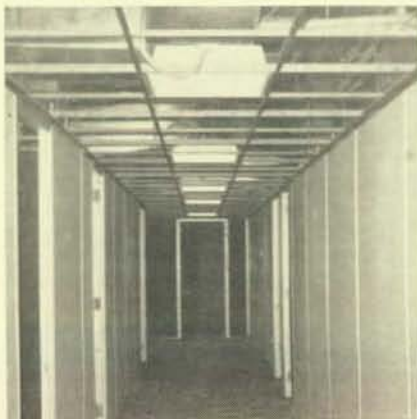
View of corridor.
