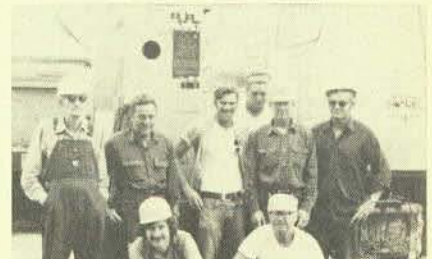
Linemen members of Local 295 employed by Power Constructors, Inc., doing outside distribution work in the Conway, Arkansas, area. Shown kneeling are, left to right, Local 346, Arlington, Tex., Brother Rickey Flatt; Local 295 Brother Dave Billings. Standing, left to right, Local 295 Brother Henry Smith; Local 108, Tampa, Fla., Brother Roy Baker; Local 295 Brothers Larry Williams, Jerry DuBose, John Simmons, Roy Williams.
