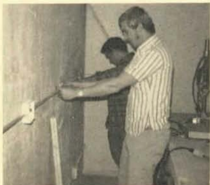
Apprentices Terry Bernhardt and John Sencenbaugh install wall outlets.
