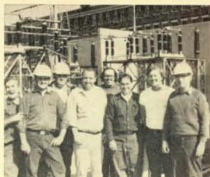
Members of Local 103, Boston, who work on the K Street Substation, in South Boston. Left to right, John Collins, Sr.; Bill Setterlund; Paul Scally of Local 104, Boston; Paul Sweeney; Frank Davey; Carmen Meo; James O'Brien; and foreman Jack McClellan.
