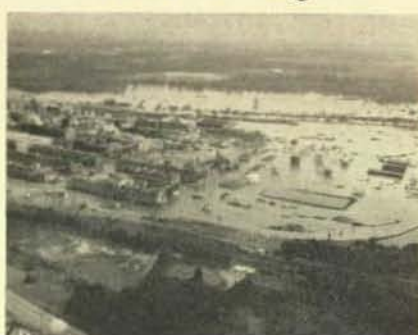
American Cyanamid's Bound Brook Plant lies idle and quiet under receding flood waters, the aftermath of Hurricane Doria, which caused untold damage and which taxed the manpower resources of Local 262.
