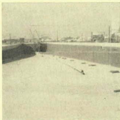
The East Side entrance and exit of the tunnels.
