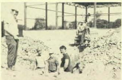
Local 305 members on the job at the new Alcoa Building.
