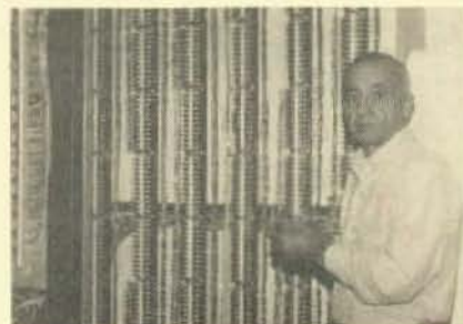
Charles Bogil, Local 68, Denver, Colo., stands by a termination panel in the Security Alarm Building of the Atomic Energy Commission's Rocky Flats Project. His outstanding work caught the attention of his co-workers, supervisors, and AEC personnel. Brother Bogil is known in the area for his neat and workman-like terminating.
