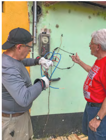
Retired Local 804 journeymen Neil Whittaker and Gerry Snyder rewire a meter at a dormitory for older students from the children's home.
