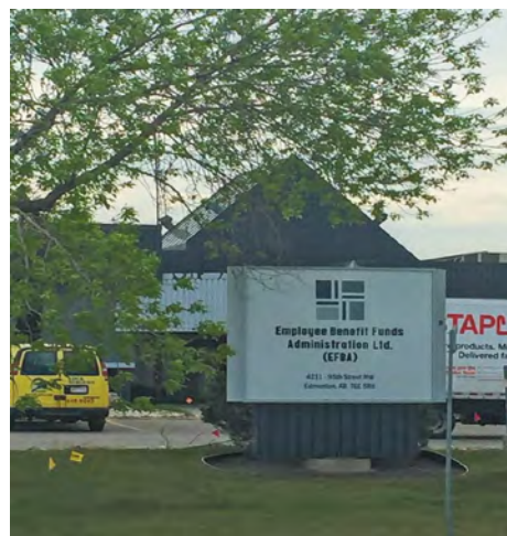
New IBEW Local 424 EBFA building.
