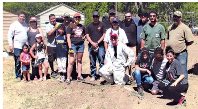
IBEW Local 611 RENEW/NextGen volunteers and assistants participated on a project to help with yard work and repairs at the home of a retired IBEW member.
