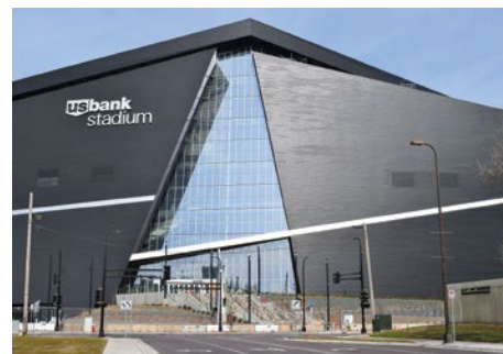
US Bank Stadium, new home of the Minnesota Vikings, constructed by IBEW Local 292 members and many other trade union workers.
