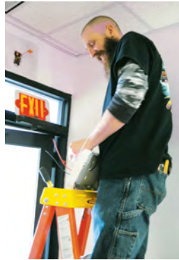
Local 673 Bro. Lloyd Brannon replaces an exit sign at union hall.
